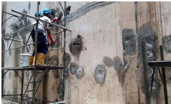
Repairs and Waterproofing Work in Progress
