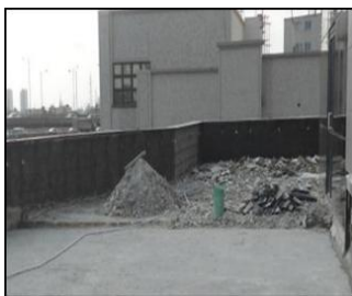
Leaking Roof Terrace with damaged Felt and Tiles
