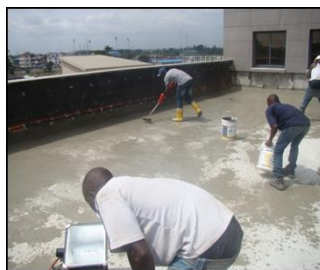
Krystol & Laticrete Surface Treatment in progress
