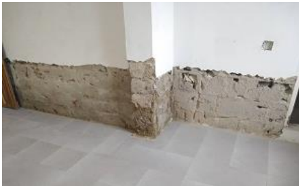
Removal and disposal of plaster
