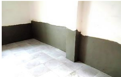
Re-plastering With KMA Treatment
