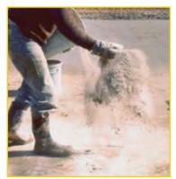
Krystol Broadcast produces a smooth finish and is used to integrally waterproof and add durability to concrete slabs that will be power-troweled during finishing:
